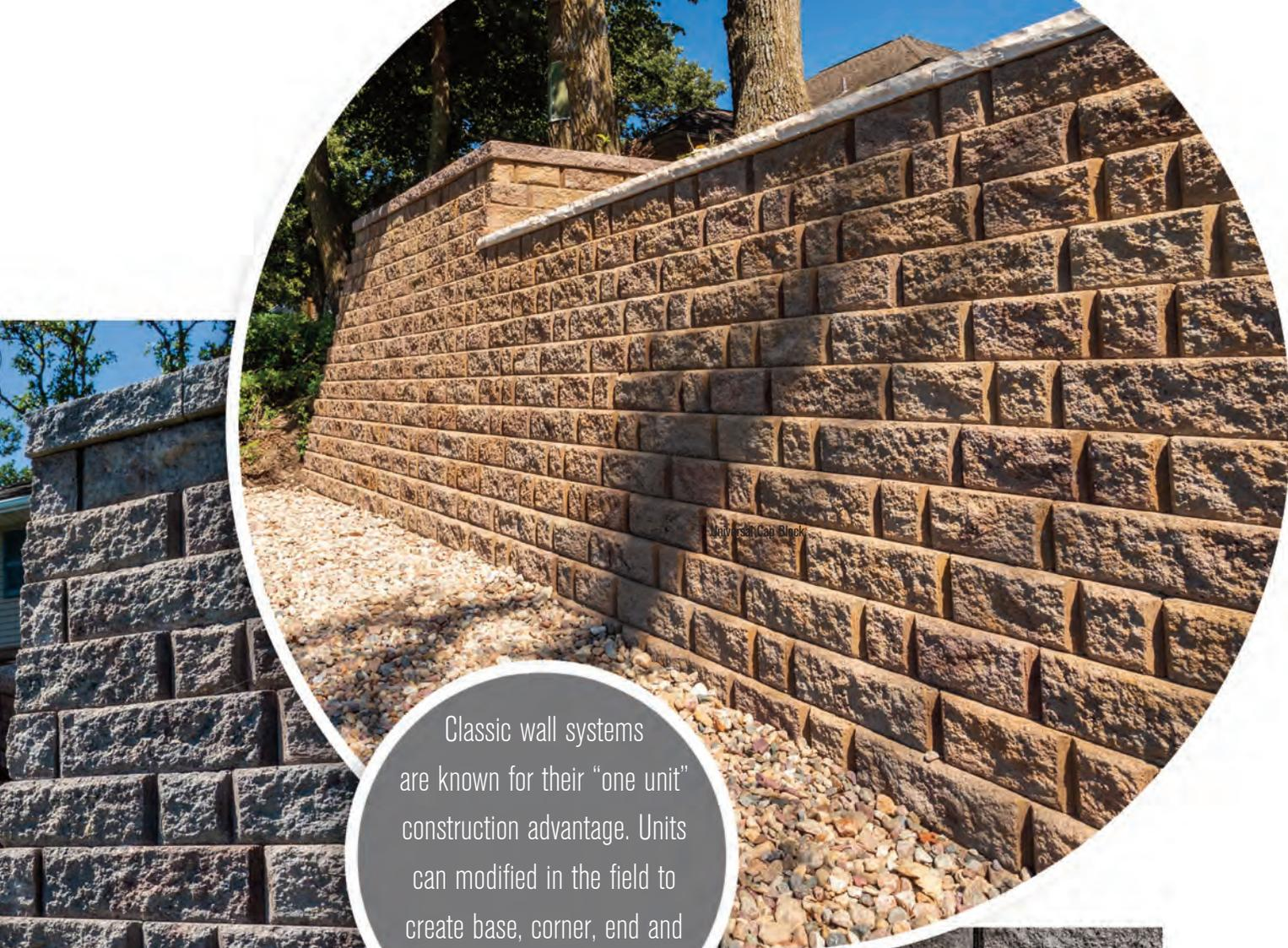
Classic wall systems are known for their “one unit” construction advantage. Units can be modified in the field to create base, corner, end and pillar blocks.
